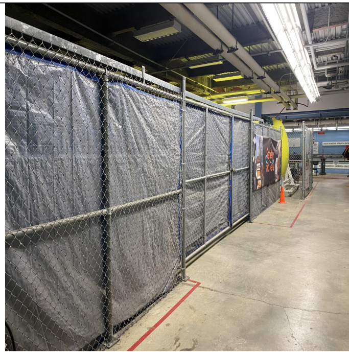
IMAGE 1: CHAIN LINK ENCLOSURE
