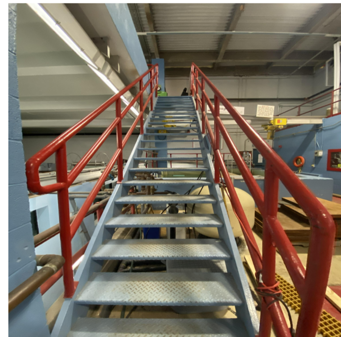
IMAGE 10: STAIRS, MEZZ ACCESS
